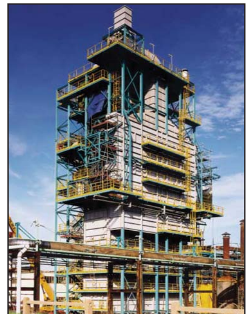
Ethylene Cracker Unit
